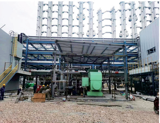
多晶硅闪蒸罐高温水余热利用（闪蒸+蒸汽压缩机） 两台串联、二级升温 High temperature water waste heat utilization of a polycrystalline silicon flash tank (flash+steam compressor) Two stages connected in series, two-stage heating
