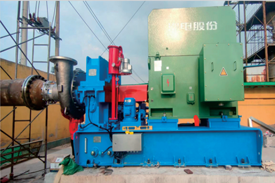
电厂末端蒸汽管道增压 Boosting of steam pipeline at the end of a thermal power plant
