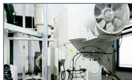
某水泥窑协同处置垃圾焚烧飞灰浸取液钠钾分离项目蒸汽压缩机 Steam compressor for collaborative disposal of waste incineration fly ash leaching solution sodium and potassium separation project in a cement kiln
