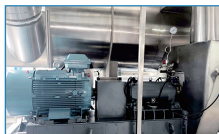
某西药生产低温浓缩项目蒸汽压缩机 Low temperature concentration of Western medicine
