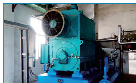
某制药废水处理蒸汽压缩机 Steam compressor for pharmaceutical wastewater treatment
