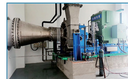
某三元前驱体废液处理项目蒸汽压缩机 Ternary precursor waste liquid treatment project
