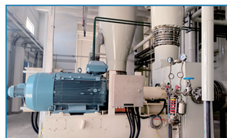
某煤矿矿井水深度处理项目蒸汽压缩机 Coal mine wastewater treatment
