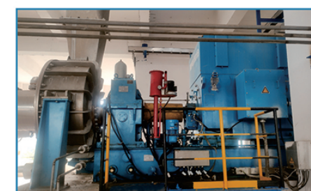
某电池新材料前驱体项目中水回用装置蒸汽压缩机 Steam compressor for water reuse device in a battery new material precursor project
