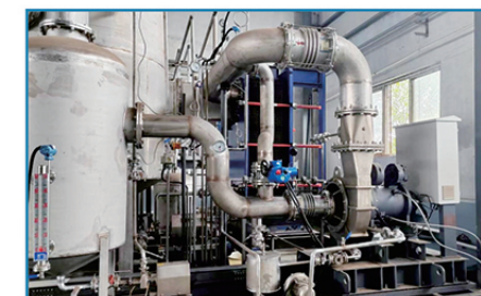
某饲料添加剂蒸发浓缩项目蒸汽压缩机 Steam compressor for a feed additive evaporation and concentration project 蒸发量：4 t/h Evaporation capacity: 4 t/h
